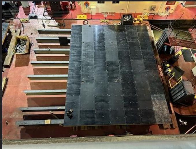
Installing Plywood on Flipped Formwork
