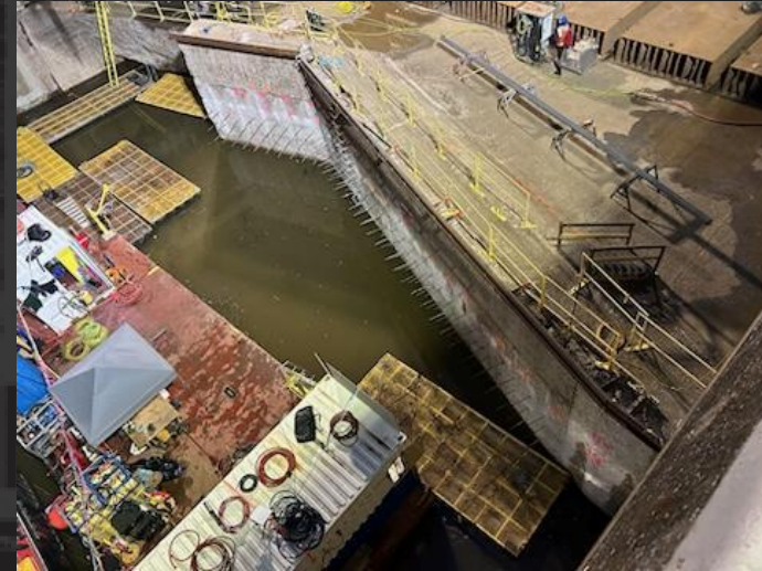
Installed Dowels in Sill Face
