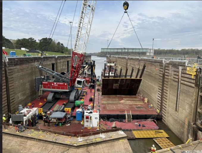
Flipping Assembled Concrete Formwork
